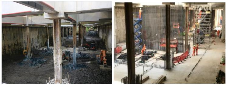
Fig.1 Excavation to B14 at Nine Elms Station
